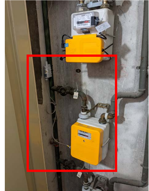
Pulse sensor for Gazpar smart meter
