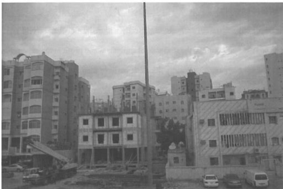
Figure 7. Construction of a new building on the 4 th ring road. Photo by the author
