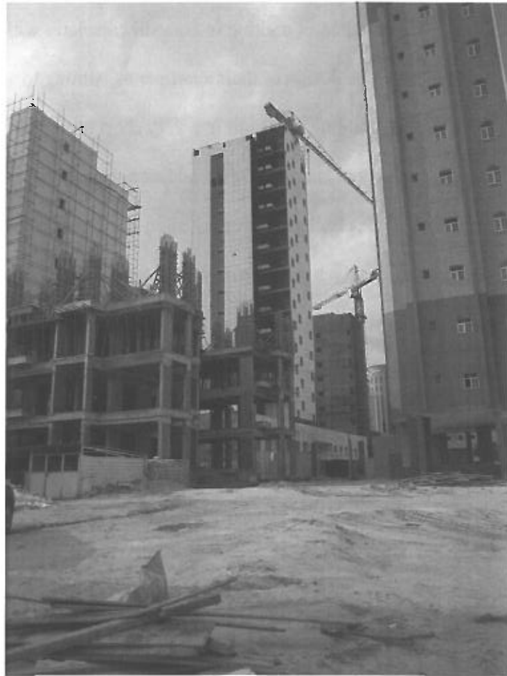
Figure 6. Buildings under construction in a Hawalli alleyway. Photo by the author
