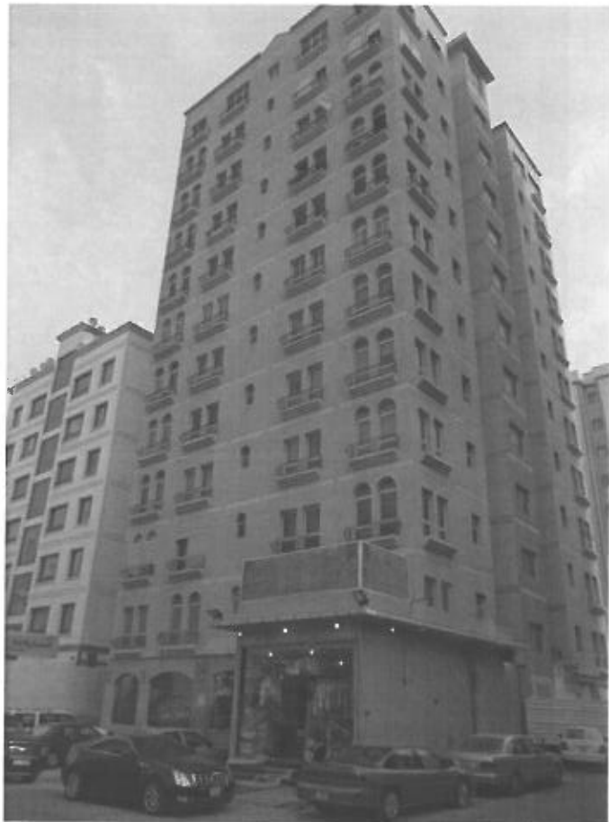
Figure 4. Huge modern complex with no enough parking spots, Hawalli. Photo by the author
