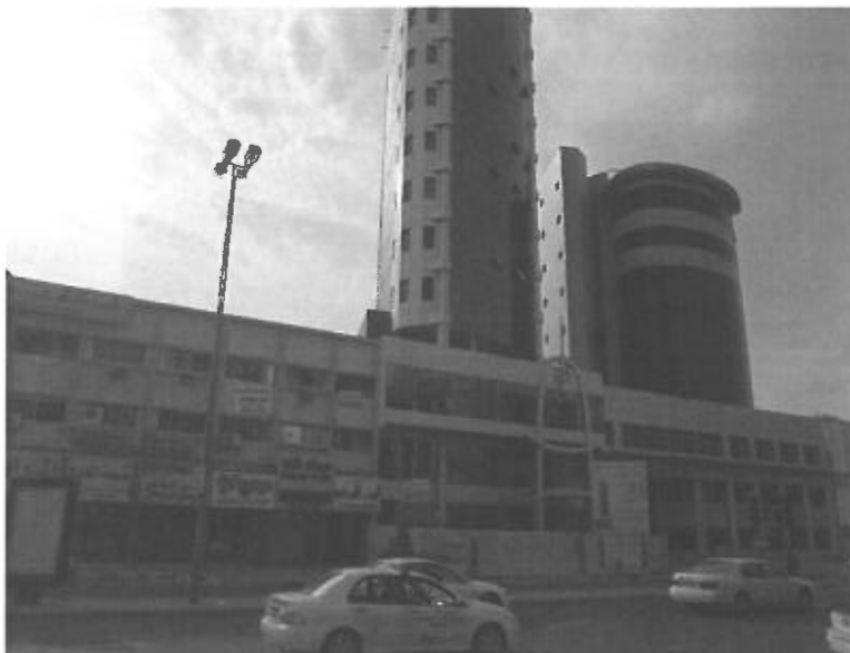
Figure 9. Demolishing the old to construct the new; creating the 'spectacle' and profit, Tunis St. Photo by the author
