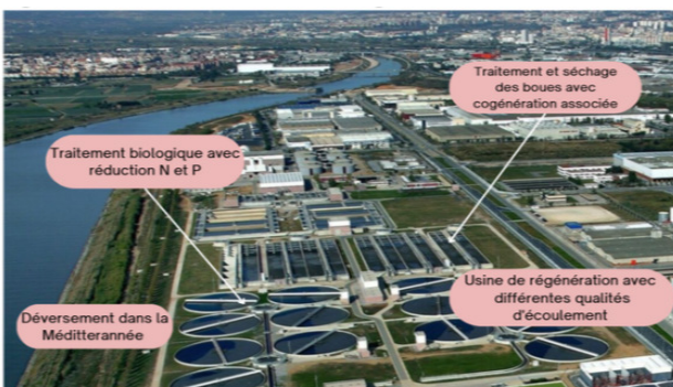
Diagram of the operation of the Bas-Llobregat wastewater treatment plant (Gullón Santos & Aguiló Martos, Niza 2009)
