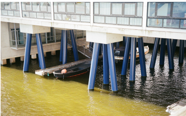
Amsterdam, IJburg district, built on a series of artificial islands to the east of the city (Urban Planning Master students, group with Altémed, 2025)
