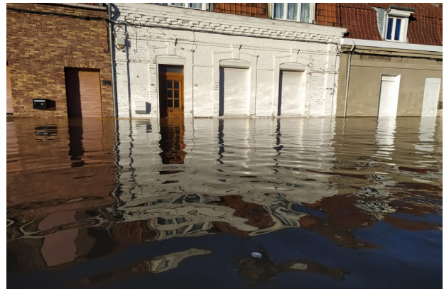
House in Arques (Nord-Pas-de-Calais) during the 2023-2024 flooding. Picture generously given by the landlord.
