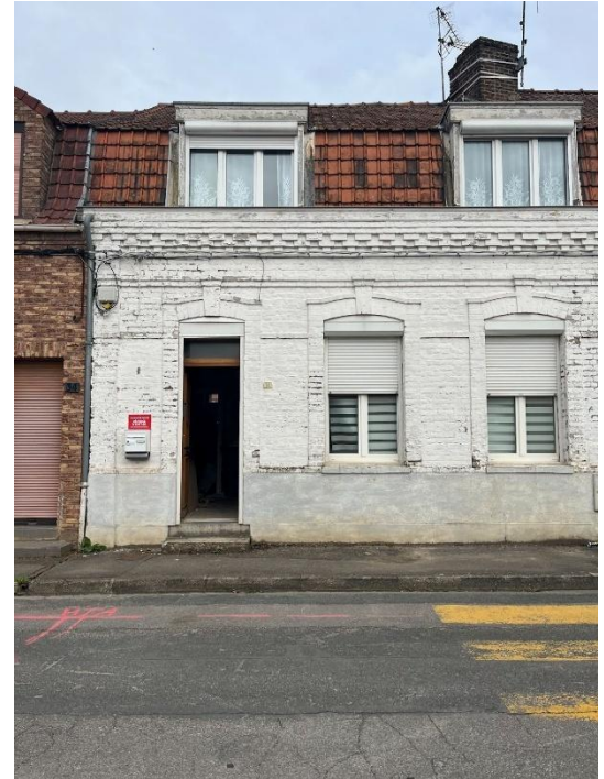
Figure 3: Photo of the same house in Arques, during our field visit, March 2025. Credit : Iris Aubé.
