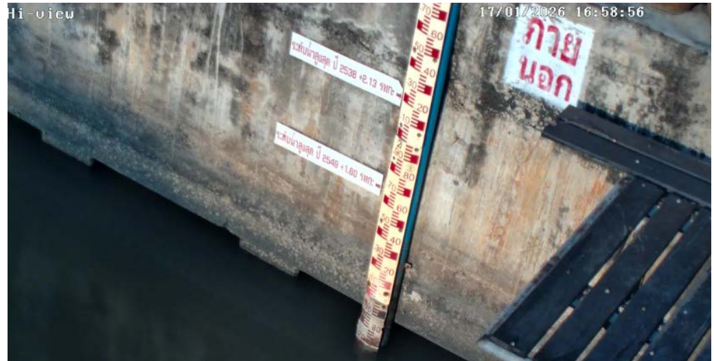
Figure 3: On-site measurements help track changing water conditions and improve early warning systems, Bangkok Metropolitan Administration, Flood Risk Locations Dashboard, 2026
