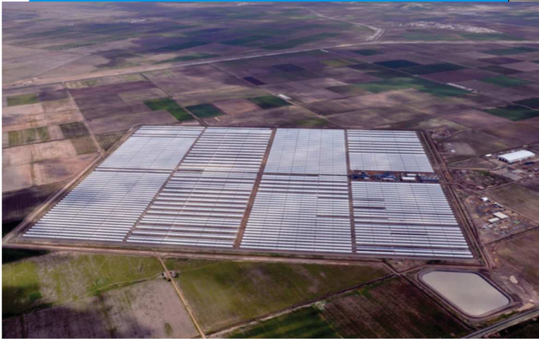
Lebrija CSP plant will be ready for grid connection on 1 January 2011. (Picture courtesy of Siemens).
