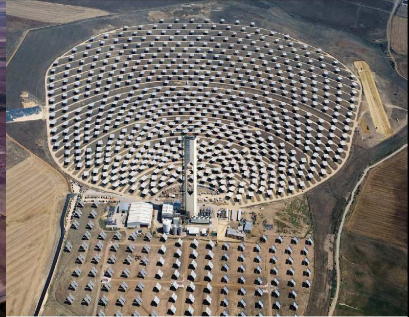
Spain's first commercial concentrating PS10 solar power tower is operating near the sunny southern Spanish city of Seville. The 11 MW solar power tower produces electricity with 624 large movable mirrors called heliostats.
