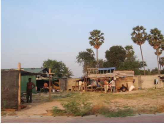
Image 19: Construction in SEZ
